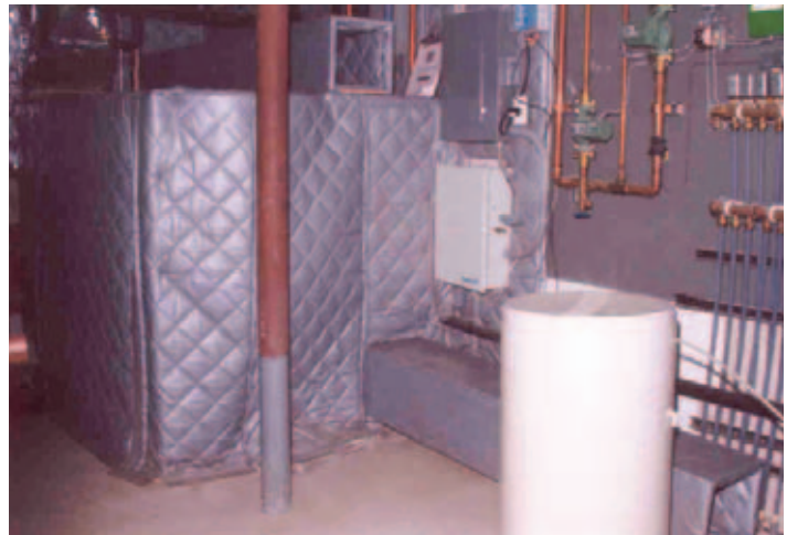
Figure 10. With basements increasingly used for living space, heating and air-conditioning noise is a growing problem. Adding acoustic controls is a good idea, but the products installed in mechanical rooms must be Class-A fire-rated.
