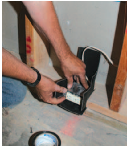
Figure 5. Electrical boxes, a common sound-leakage point, are easy to seal with site-built enclosures (above left) or acoustic barriers like mass-loaded-vinyl. Here, a worker folds and tapes a precut piece of mass-loaded vinyl around a single-gang box (above right). After the drywall is hung, each box should be sealed around the perimeter with acoustic sealant. When possible, outlets on opposite sides of a wall should be offset by at least three stud cavities.
