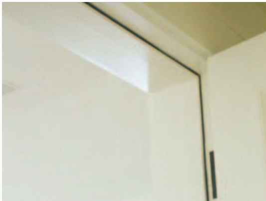
Figure 9. Without a proper door, home theaters can be a source of irritation to family members trying to study or sleep. Any door separating a media room from the rest of the house should have a solid core, an acoustic sweep, and good weather stripping. An acoustically rated model is preferable.
