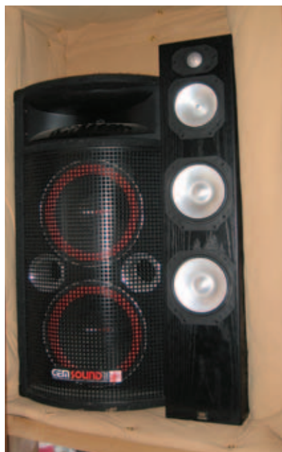
Figure 2. To control low-frequency structure-borne noise, the sound source must be decoupled from the framing. That was accomplished here by installing a layer of foam-backed, mass-loaded vinyl called NoiseOut2 under and behind the speaker. The material can also be used with subwoofers, hvac equipment, and other low-frequency sound sources.
