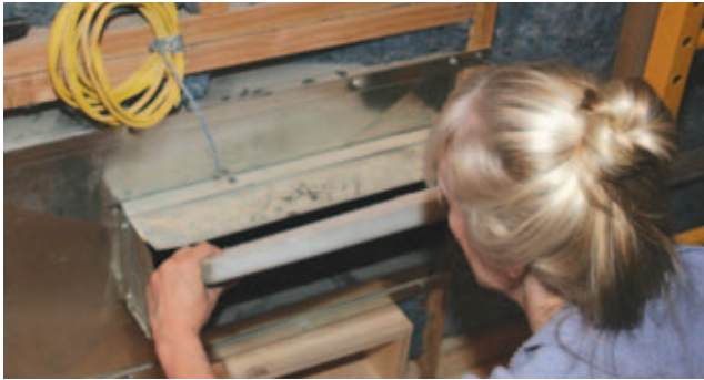
Figure 7. Preventing ducts from spreading sound throughout the house is a two-step process. First, fire-rated acoustic foam or fiberglass duct liner is installed on the ducts' interior to deaden any sound that gets inside (above); next, the ducts' exterior is wrapped (right), which ensures that very little sound will penetrate in the first place. Both steps are especially important in basement home theaters, which often have many ducts in the ceiling.
