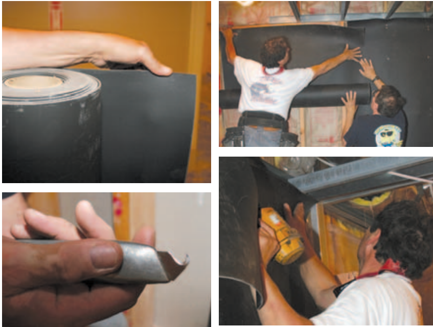
Figure 1. Mass-loaded vinyl reduces sound transmission to adjacent spaces better than multiple drywall layers and resilient channels do. The 54-inch-wide rolls (top left) are installed over the framing (top right) and lapped 6 inches between studs or joists. Cuts are made with a hook-blade utility knife (above left) and the material is fastened with a pneumatic roofing nailer (above right).
