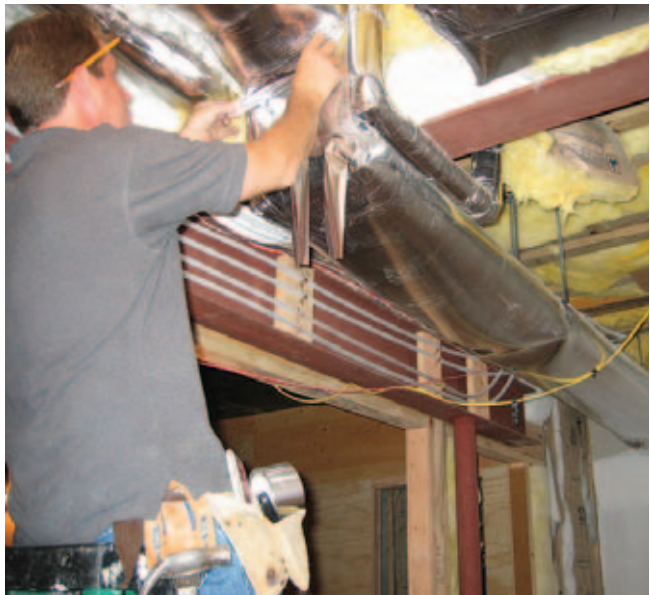
Figure 7. Preventing ducts from spreading sound throughout the house is a two-step process. First, fire-rated acoustic foam or fiberglass duct liner is installed on the ducts' interior to deaden any sound that gets inside (above); next, the ducts' exterior is wrapped (right), which ensures that very little sound will penetrate in the first place. Both steps are especially important in basement home theaters, which often have many ducts in the ceiling.
